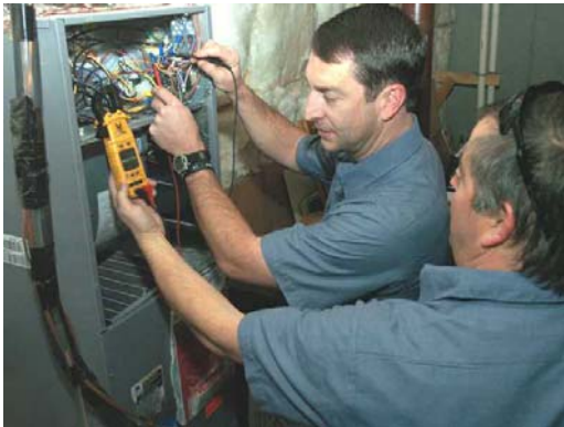
Todd Wilson gets some help servicing a heat pump from Scott Holland. Wilson will be sworn in tonight as an Oakwood City Council member.
